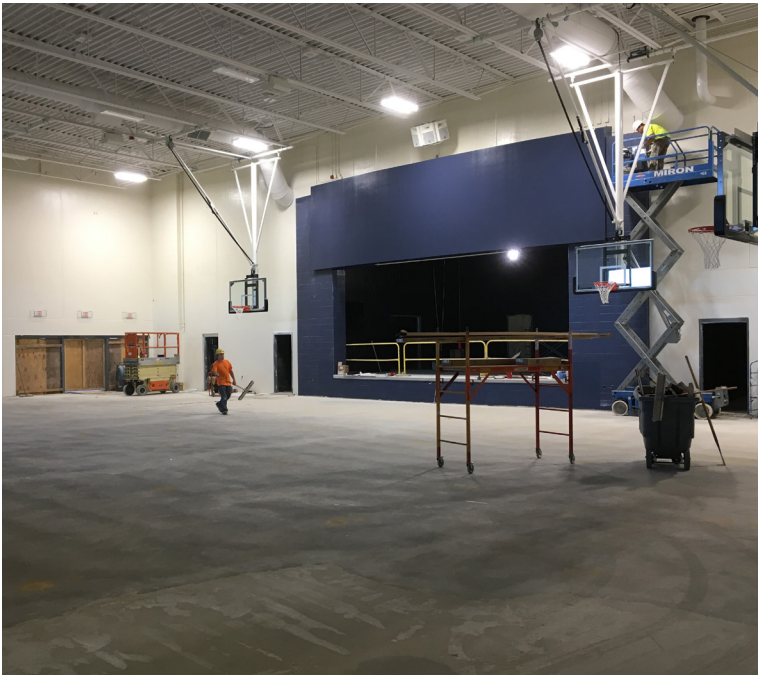
Allenton - gymnasium painting touch-ups; wood floors up next
