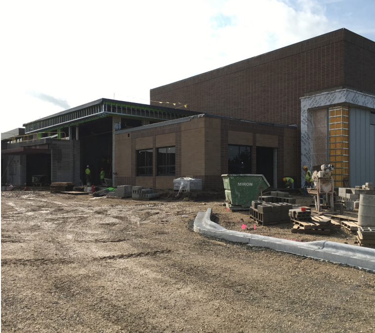
Allenton - community room windows installed; main entry progress
