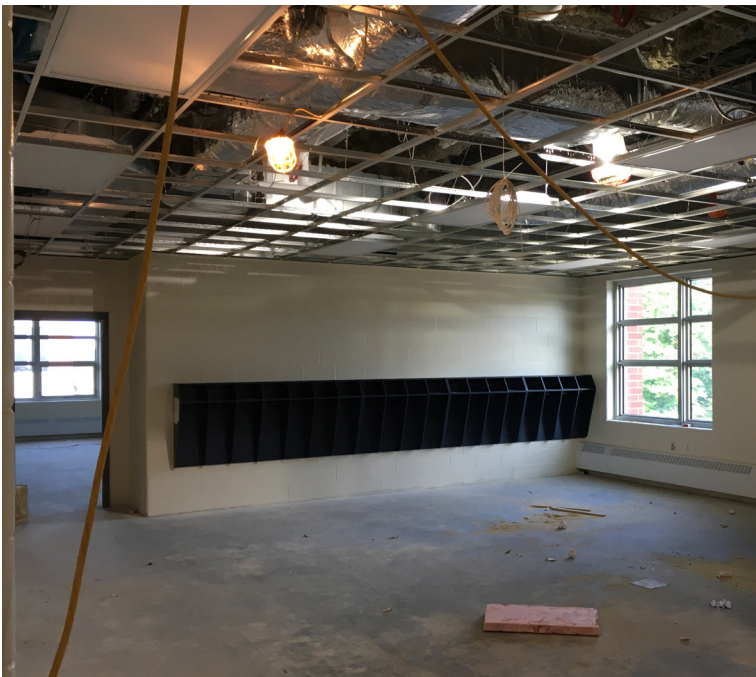
Addison - cubbies installed in second floor resource space
