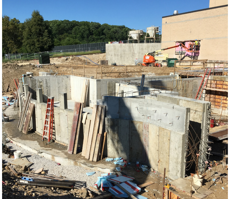
Auditorium - orchestra pit walls complete; formwork being removed
