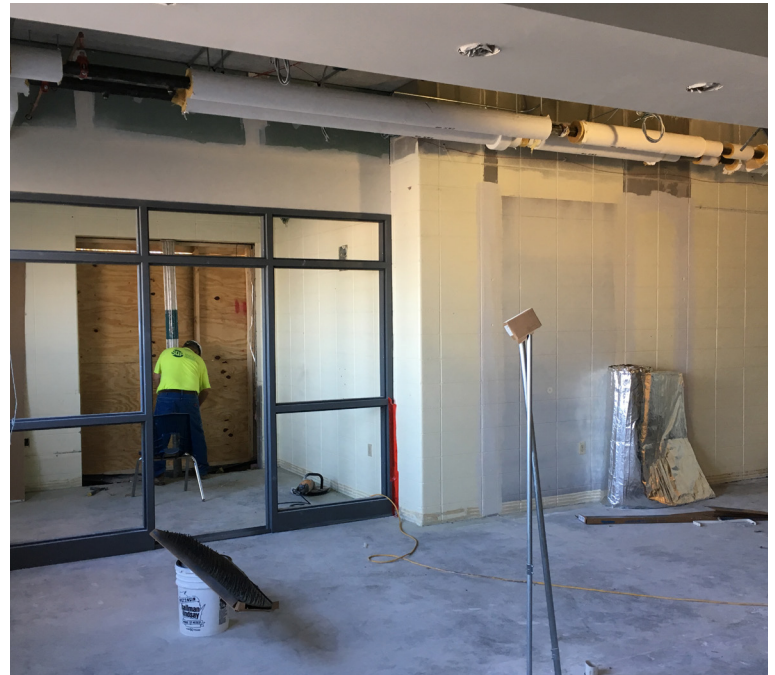
Slinger HS - view of new visitor entry from renovated main office
