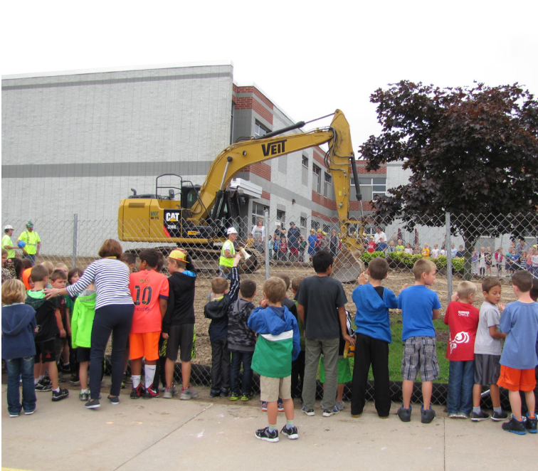
Addison - large crowd at student groundbreaking event
