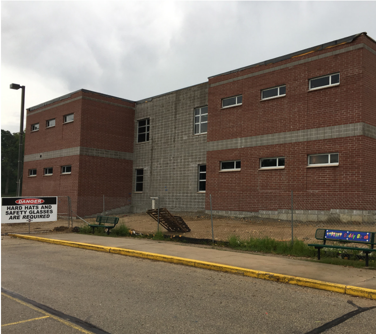
Addison - exterior brick complete and windows installed
