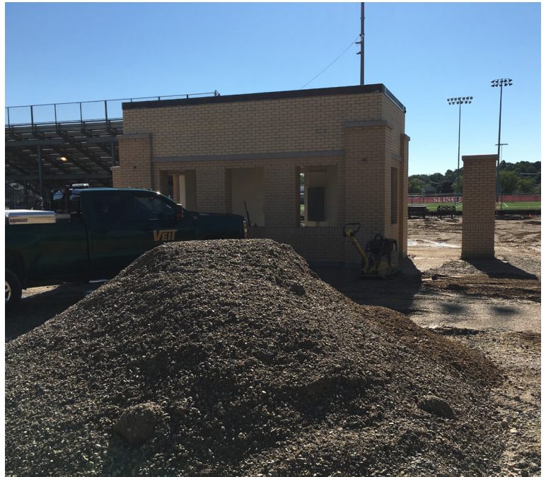
Concessions - ticket booth behind (temporary) gravel pile
