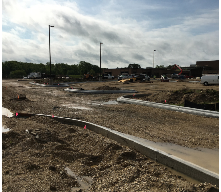
Allenton - new parking lot ready for asphalt; light poles installed
