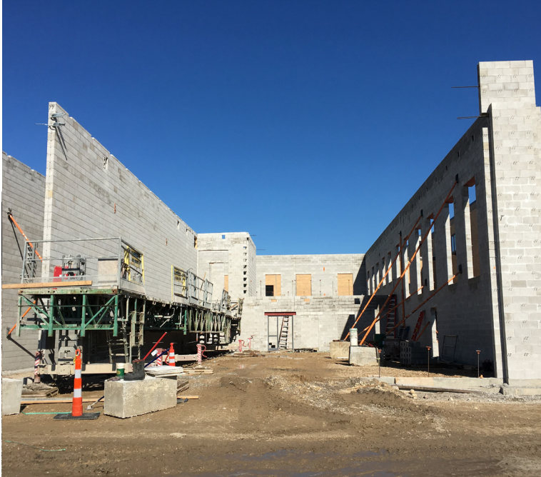
Auditorium - three walls of the band room complete; roof structure next
