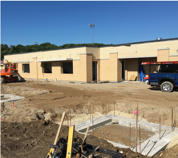
Concessions - plaza seat walls and canopy installation are in progress
