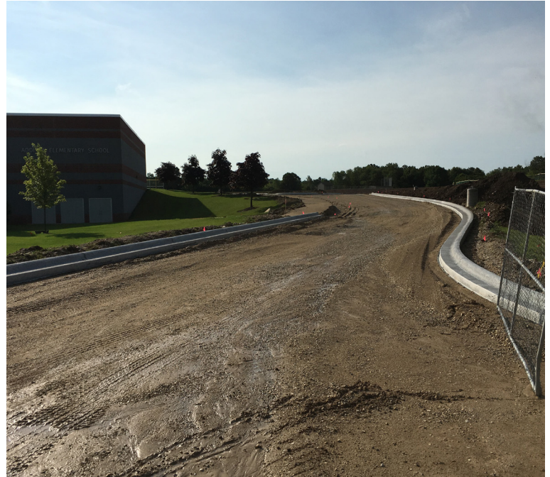
Addison - drive to expanded parking ready for asphalt
