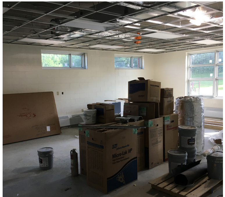
Addison - plumbing and electrical scope almost complete
