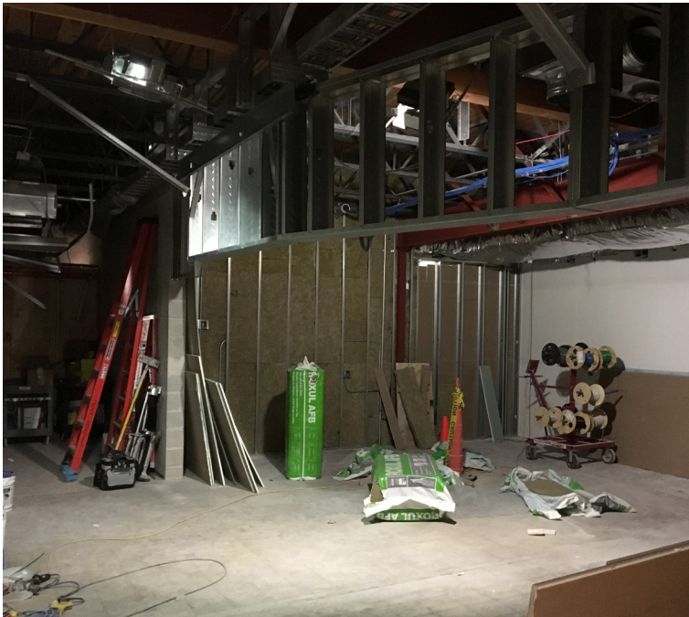
Slinger HS - The Rookery's future home; windows/doors coming soon
